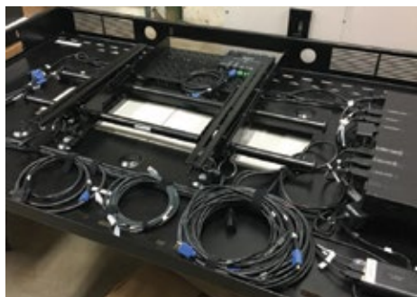
Pre-built in our assembly facility
