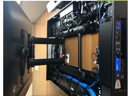
Easily serviced with the display in place
